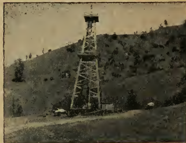
Well No. 4 now down about 900 feet. Pay oil expected soon.
